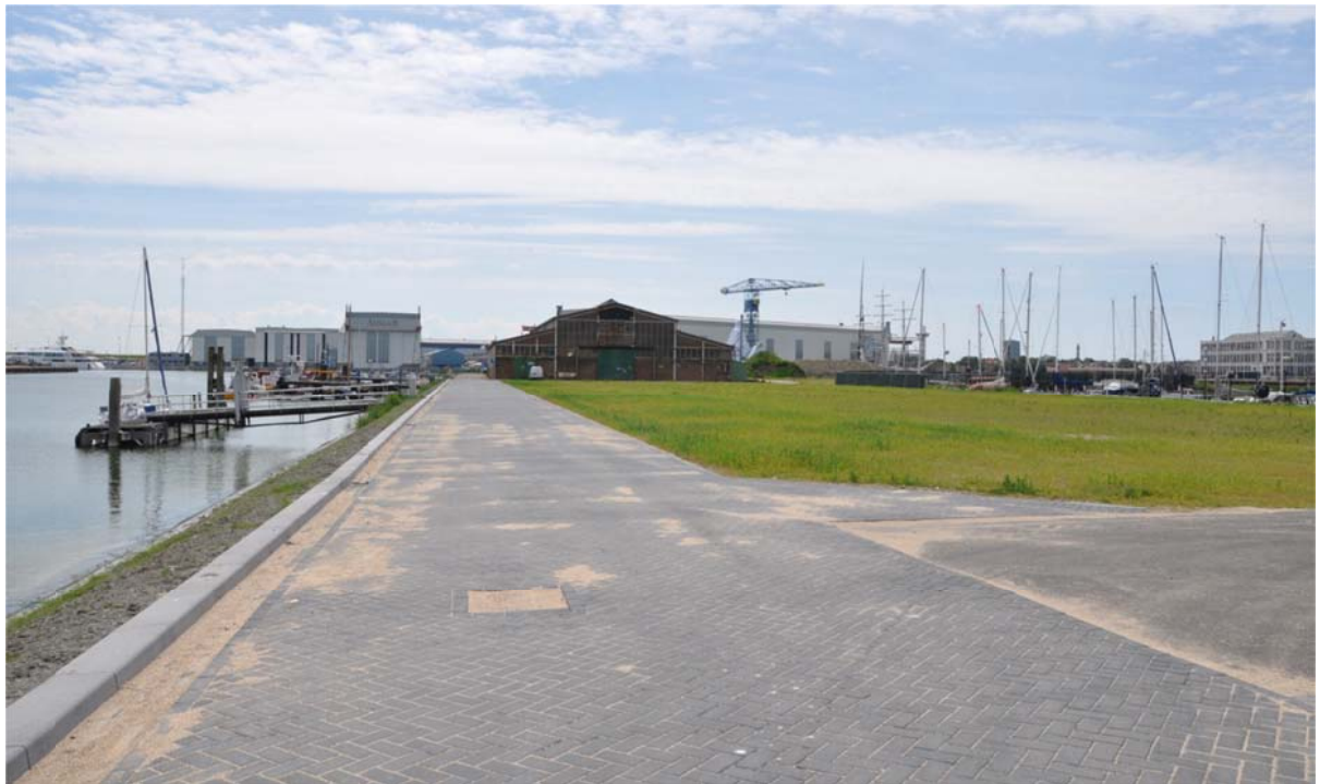
Situation at Flushing harbour (June 2014) with rebuilt access road and prepared project area
