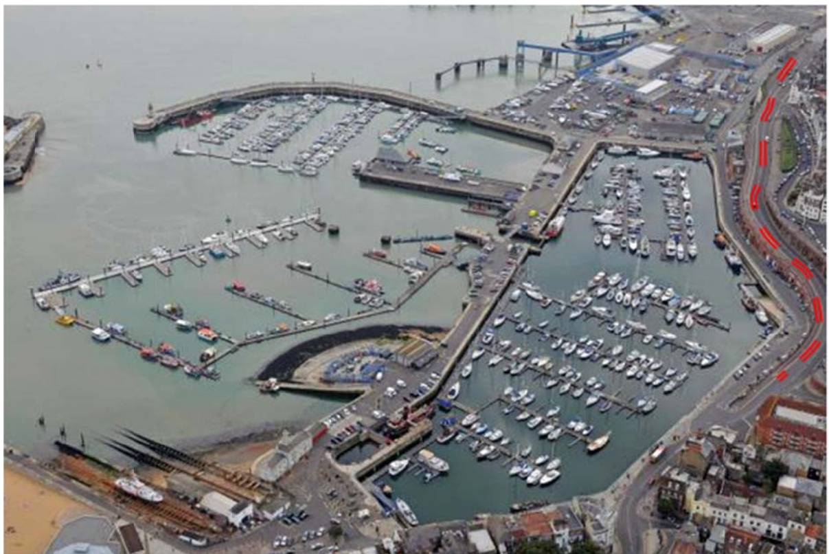
Ramsgate Harbour with the location of the Military Road Arches
