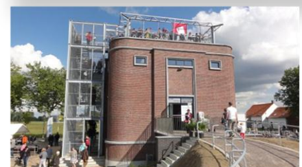
OPENING OF THE EDUCATIONAL WATER TOWER
