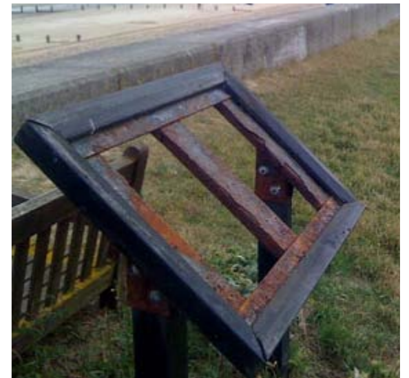
Worn, vandalised and redundant.
